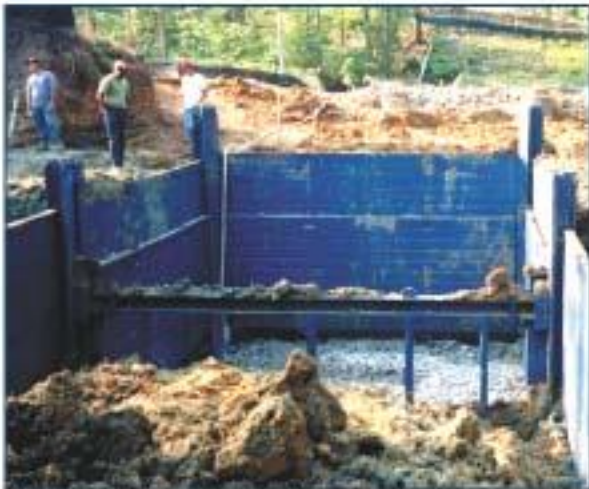
GME/E+S Modular Slide Rail System used for a pit application.
