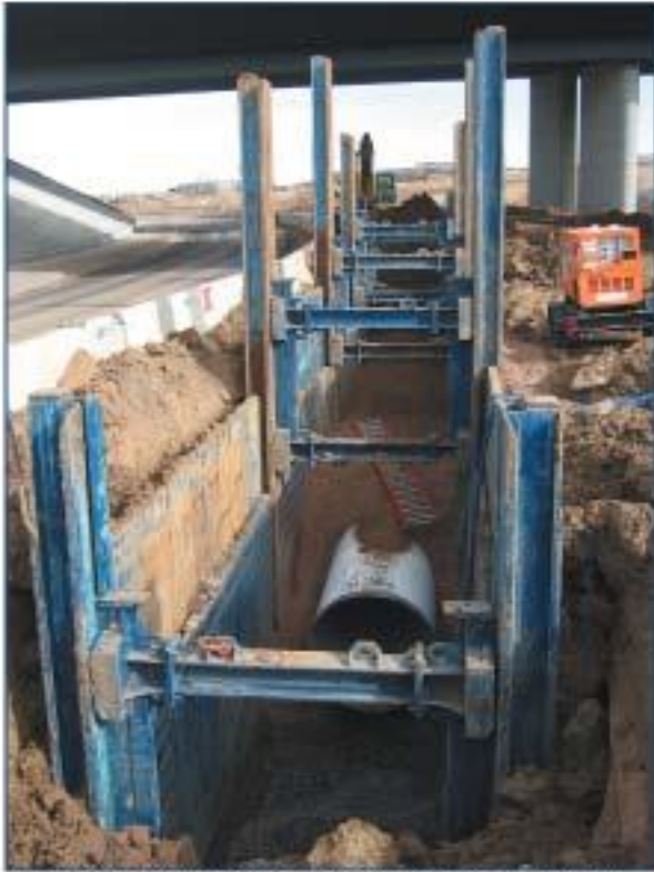
GME/E+S Modular Slide Rail System in a linear application.
